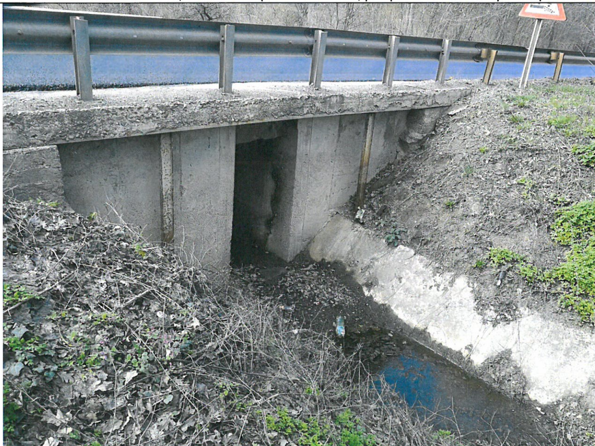
Foto 16: Drumul National DN 28, km 18+416 – podet transversal; timpan improvizat;
