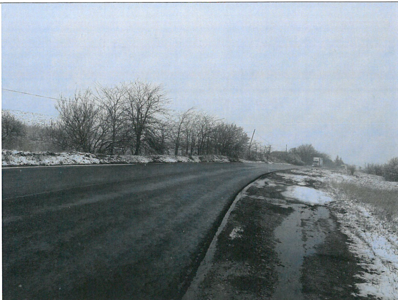
Foto 20: Drumul National DN 28, km 20+200 – lucrari recente de asternere a mixturii asfaltice.
