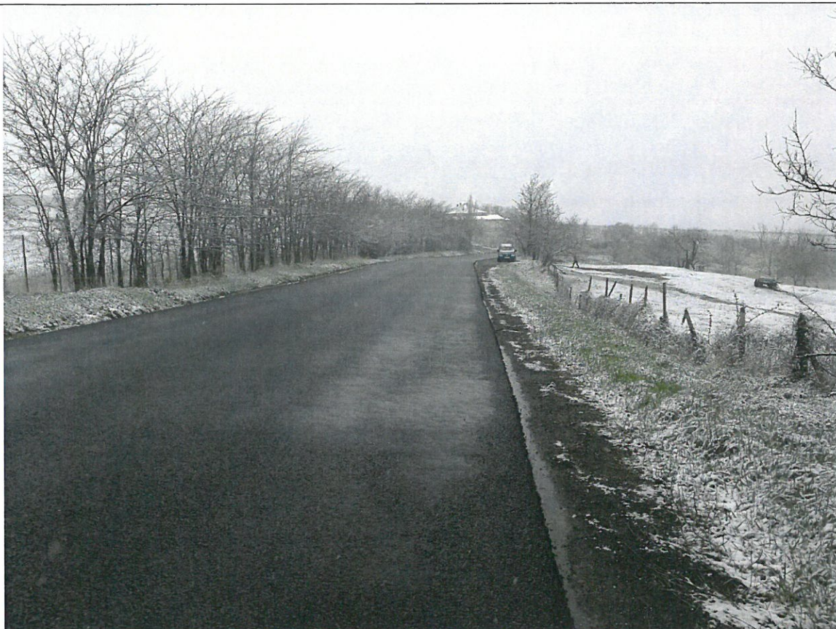
Foto 3: Drumul National DN 28, km 19+725 – acostament in pamant; taluz de rambleu inierbat.
