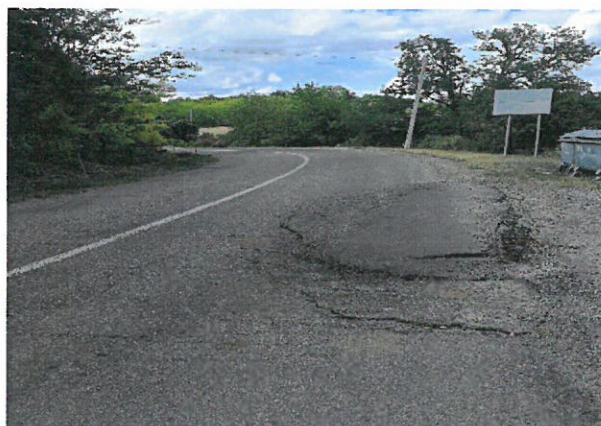
Foto 128: Drumul National DN 24C, km 106+000 – 106+663; 2 benzi de circulatie; imbracaminte asfaltica in stare rea.
