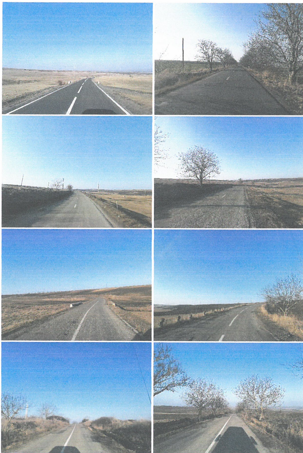
Fig. 9. Sector de drum investigat geotehnic
