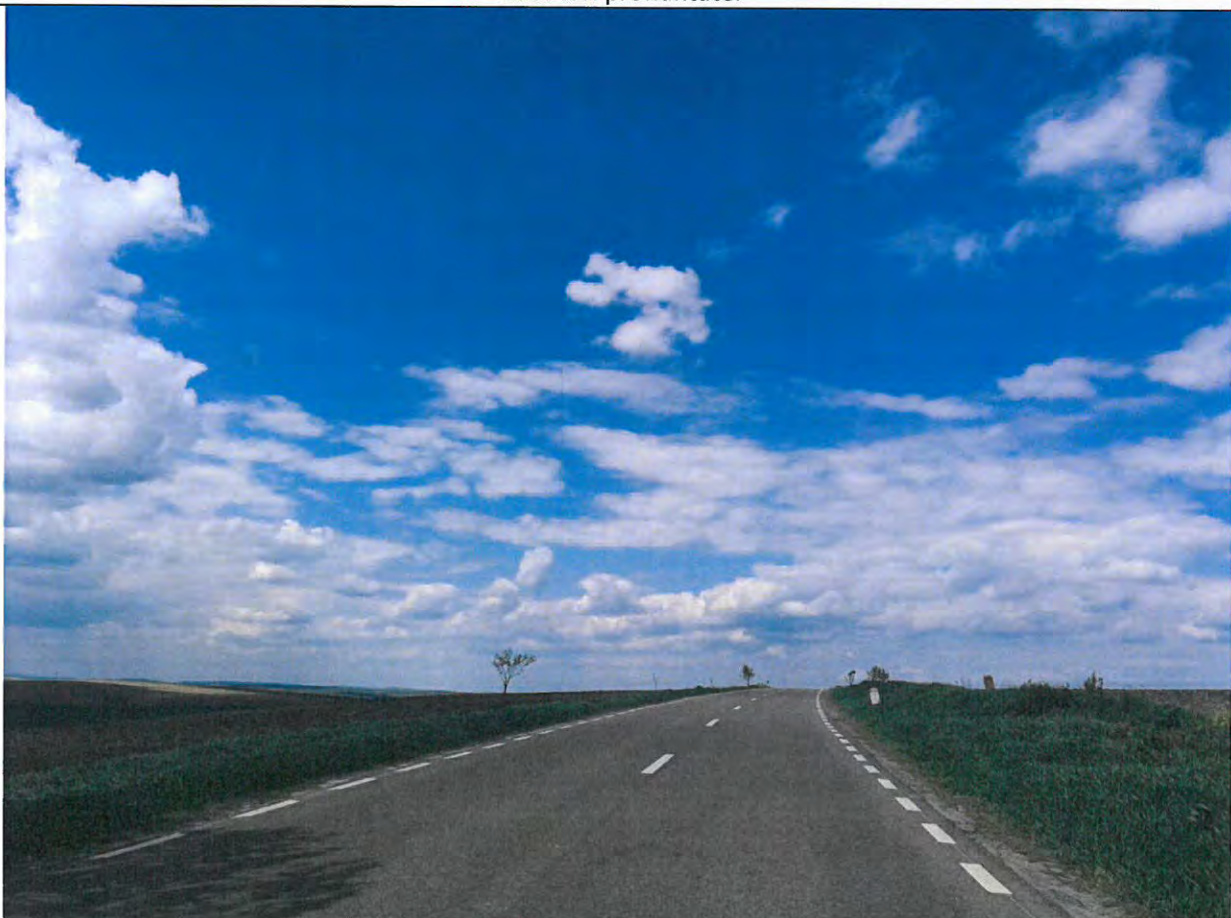
Foto 56: Drumul National DN 29, km 57+000 - 58+000 – Cale de rulare aflata intr-o stare optima de exploatare.
