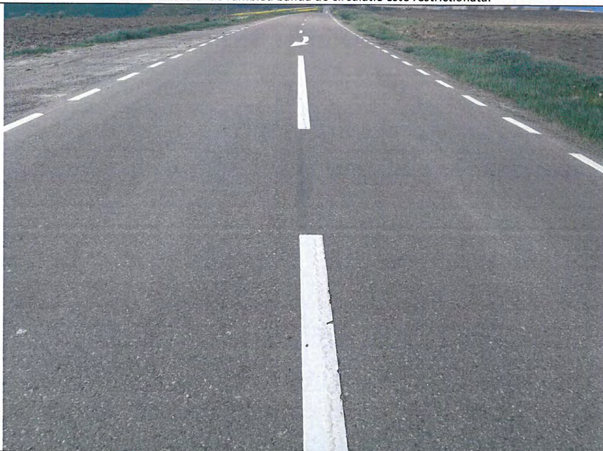
Foto 60: Drumul National DN 29, km 58+000 - 59+000 – Cale de rulare aflata intr-o stare optima de exploatare.
