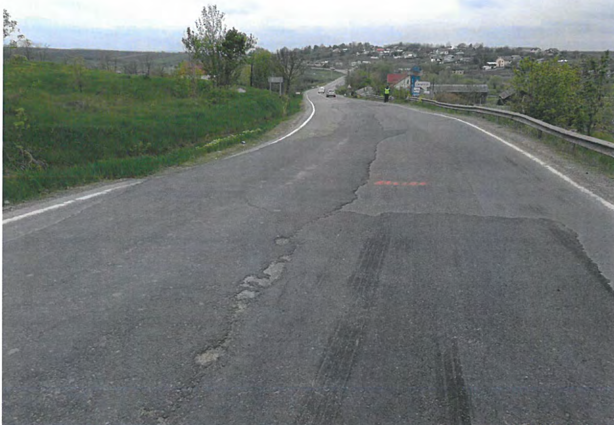
Foto 23: Drumul National DN 29B, km 11+000 -12+000 – Sector de drum cu denivelari si tasari accentuate
