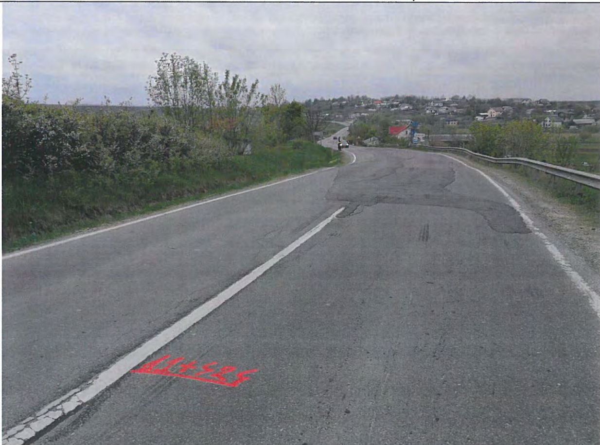
Foto 22: Drumul National DN 29B, km 11+000 -12+000 – Sector de drum cu denivelari si tasari accentuate
