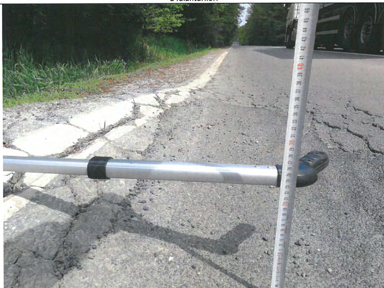
Foto 54: Drumul National DN 29B, km 19+000 -20+000 – Refulari de margine, tasari locale.
