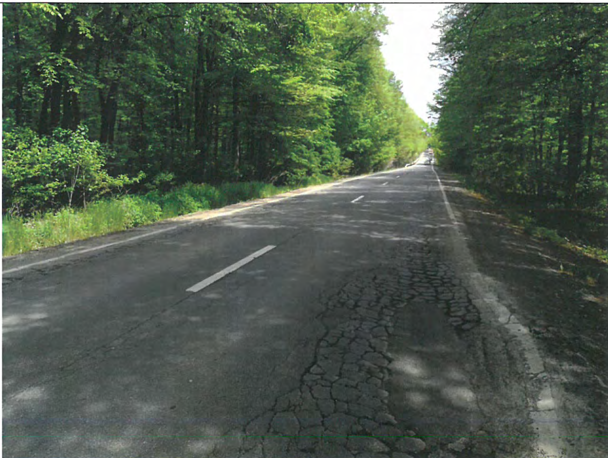
Foto 55: Drumul National DN 29B, km 19+000 -20+000 – Faiantari propuntate, refulari de margine.
